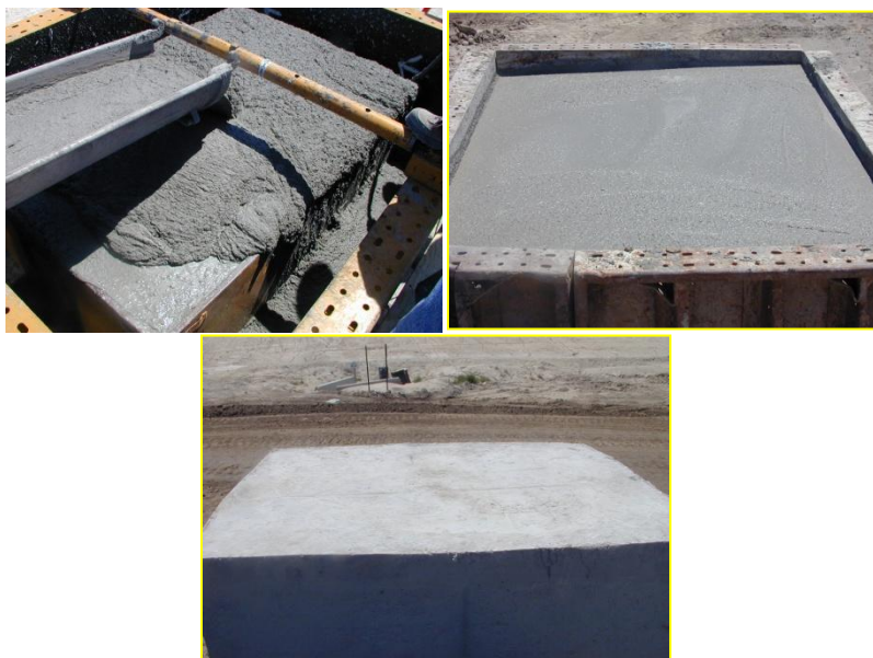
Figure 3-1. In-Cell Macroencapsulation of RCRA Hazardous Debris
