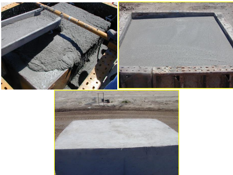
Figure 3-1. Macroencapsulation of RCRA Hazardous Debris
